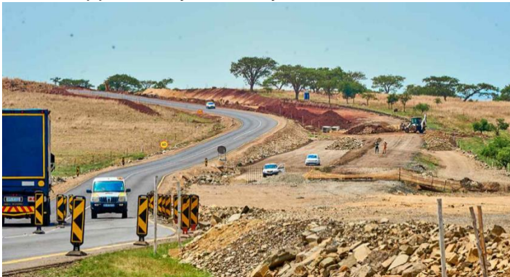
N11 ROAD CONSTRUCTION
